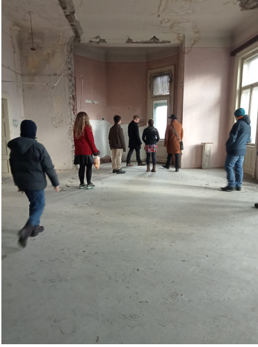
This is the "before" picture of our sanctuary in Brasov Romania before renovations began.
