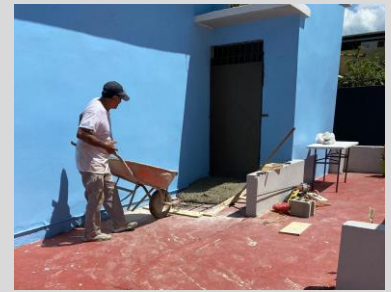
Creating ramps into the buildings.
