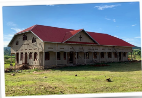
The completed roof of the LTCU chapel and multi-purpose building!
